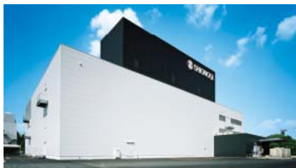
Solid formulation manufacturing and packaging facility at the Settsu Plant
